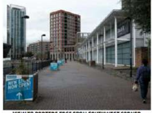
VIEW TO PORTERS EDGE FROM SOUTHWEST CORNER
