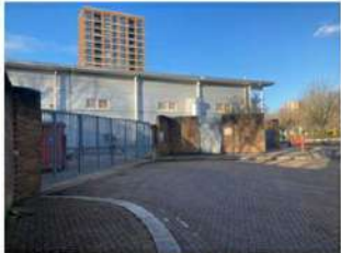
EXISTING SERVICING ACCESS
