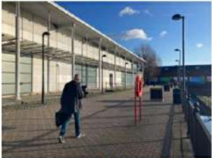
EXISTING BUILDING FROM DOCK EDGE
